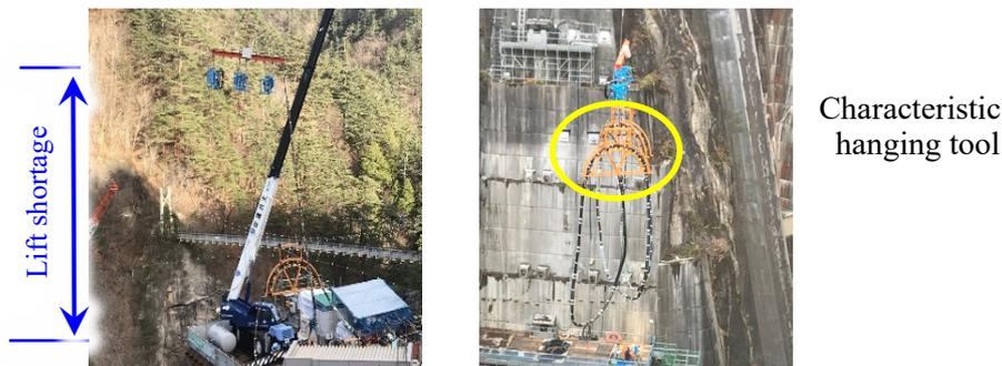
Figure 14. Tendon transport lifting tool
