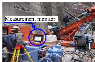
a. Drilling situation by ground exploration technology      b. Measurement circumstance of hole bending
