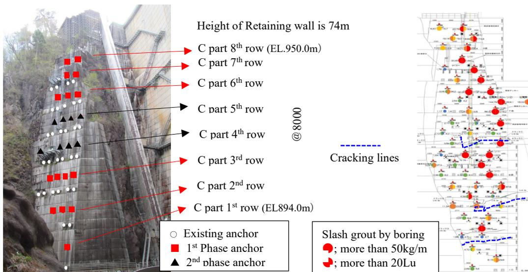
Figure 8. Front view of Right bank C part anchors, crack lines and quantity of grout injection
