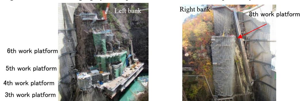
Figure 9. Large-scale Staging by work platforms on the left bank and right bank
