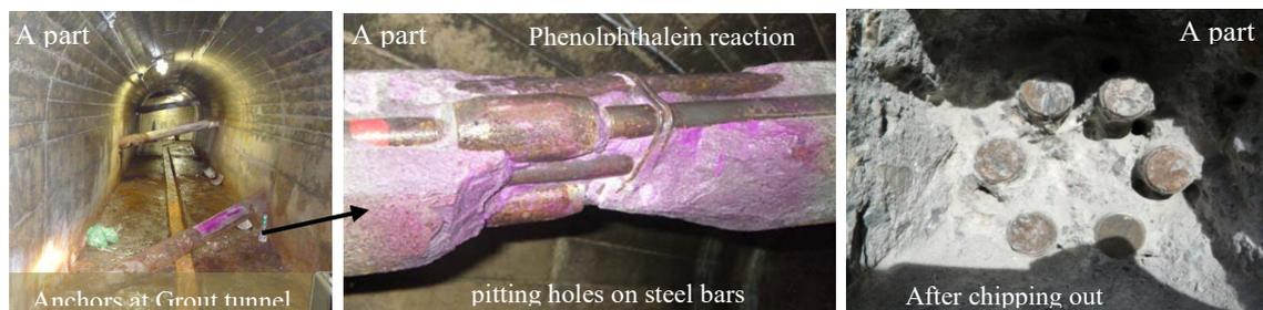
Figure 5. Pitting corrosion on a tendon at Grout tunnel and surface looks in an existing anchor
