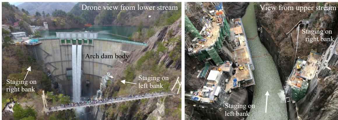
Figure 3. Situation of Kawamata Dam under the renewal works in 2019
