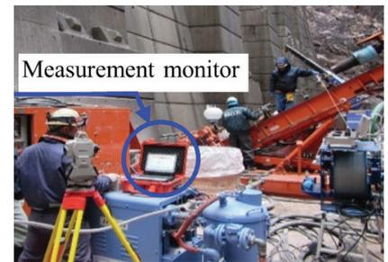
The centralized data management was performed using CIM (Construction Information Modeling) by ground exploration technology, borehole wall observation and so on. It achieved high-accuracy drilling by reflecting the drilling data. Eventually, it enabled more accurate drilling to avoid interference with other underground structures.
